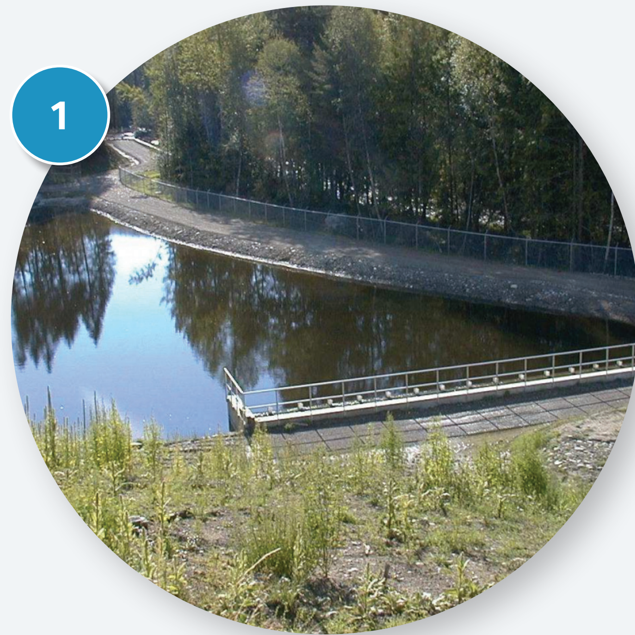
Automated Headgates and Grit Pond
