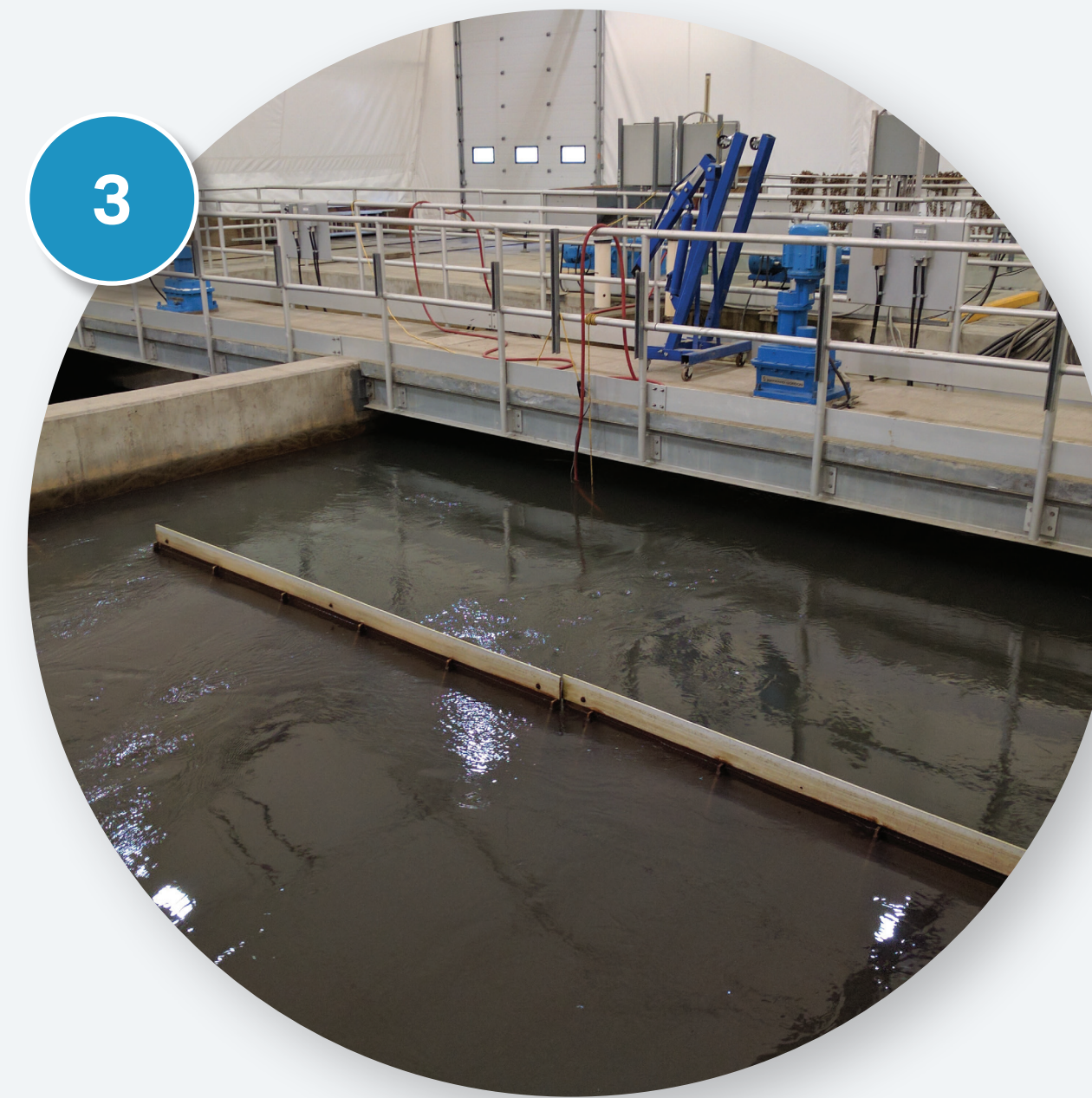
Rapid Mix and Floc Tanks
