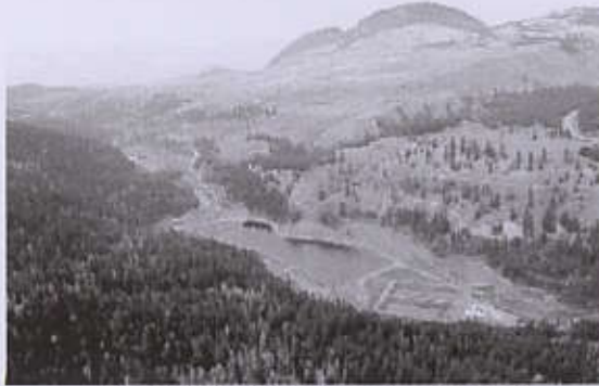
(An aerial view of BMID's Water Treatment Plant.)
