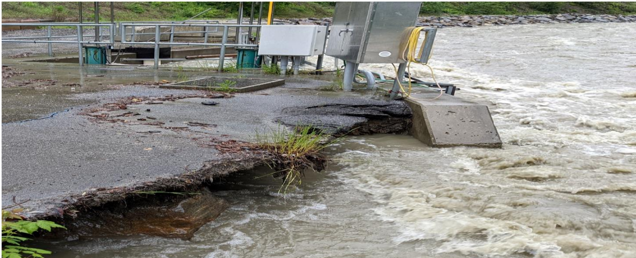
Bank erosion at Mission Creek Headgates in June 2022
