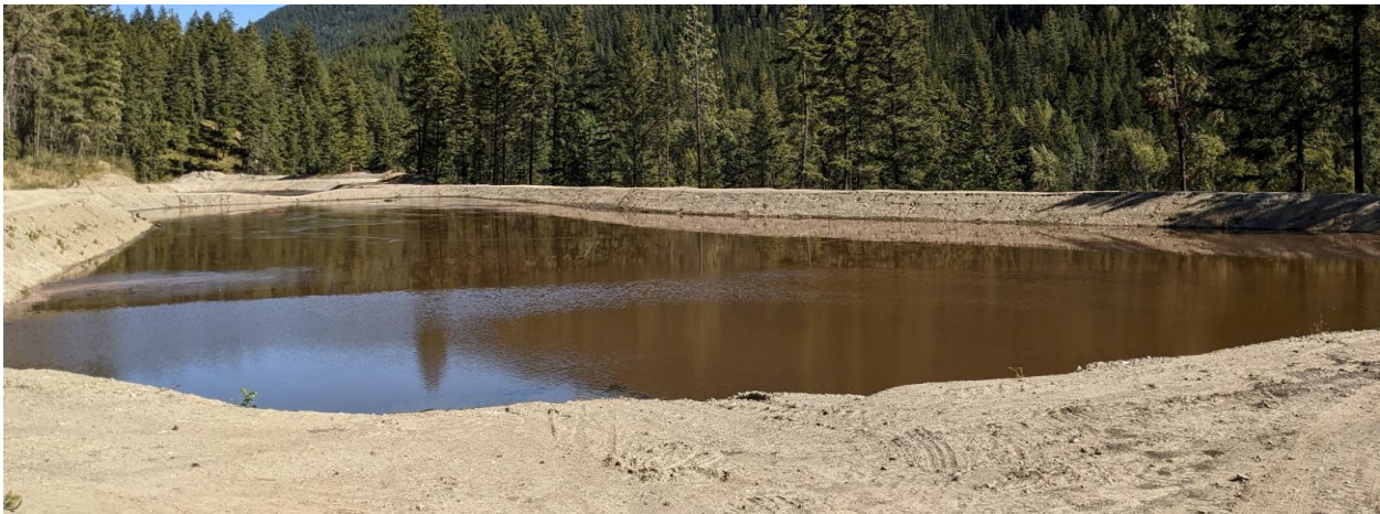
New Sludge Drying Lagoons
