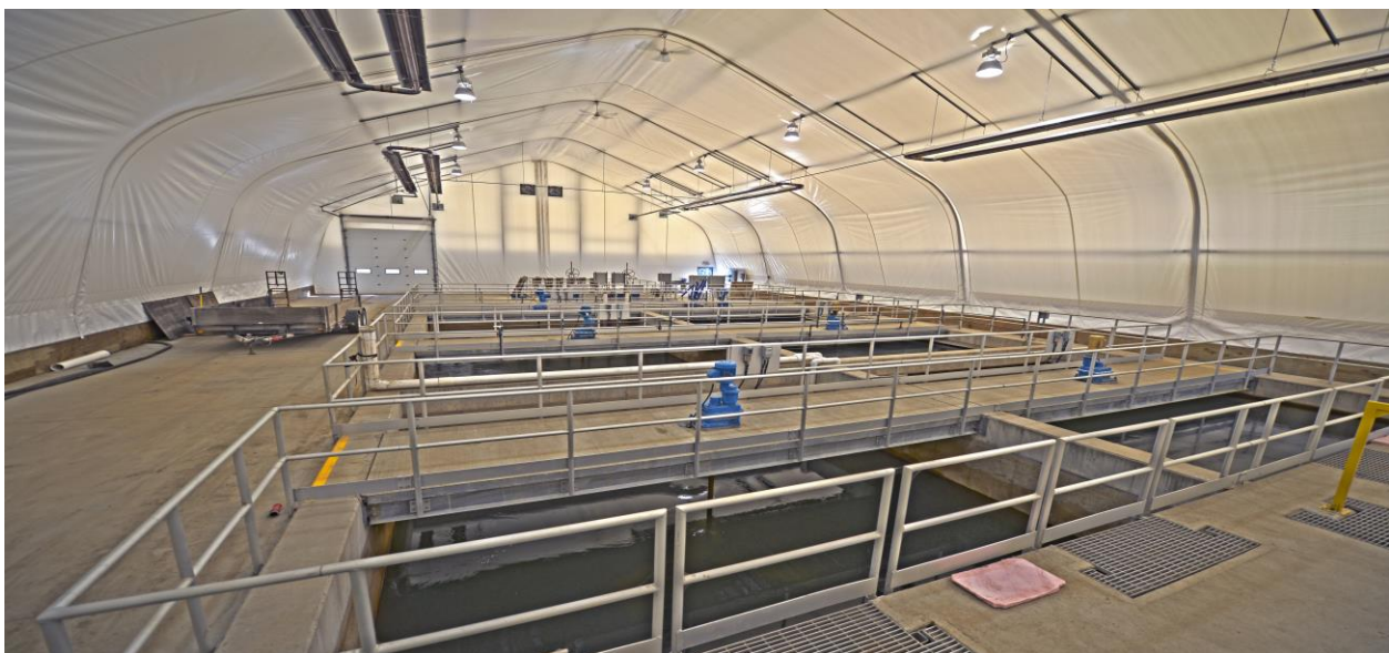
Flocculators at the Water Treatment Plant
