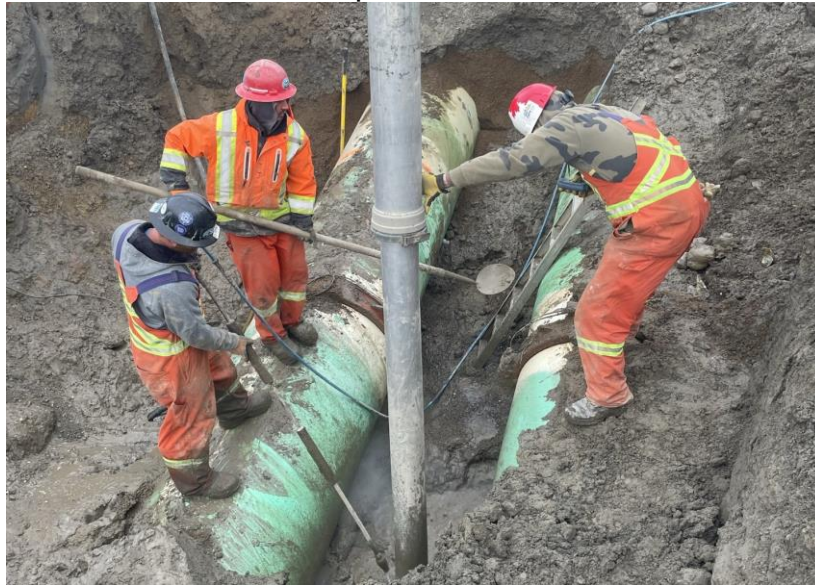
1050mm Transmission Main repair
