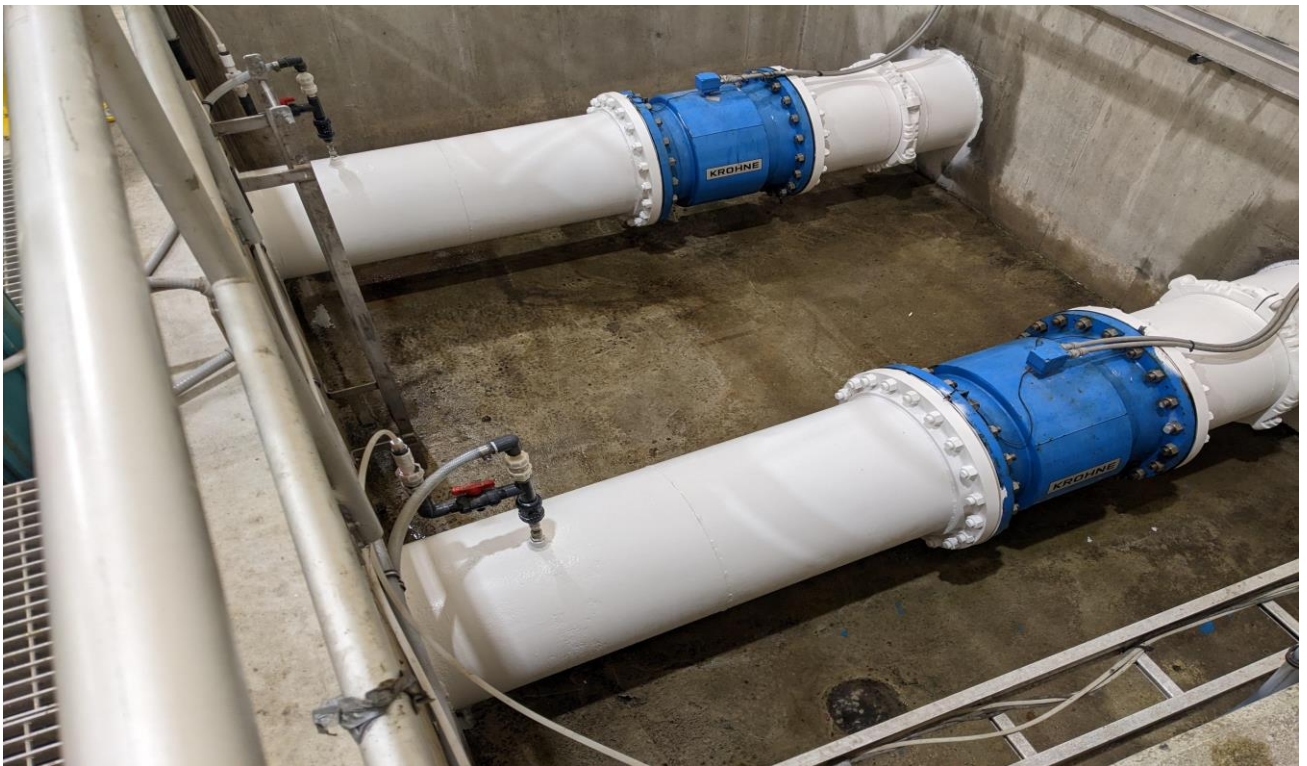
600mm steel pipe after sand-blasting and epoxy coating in meter chamber
