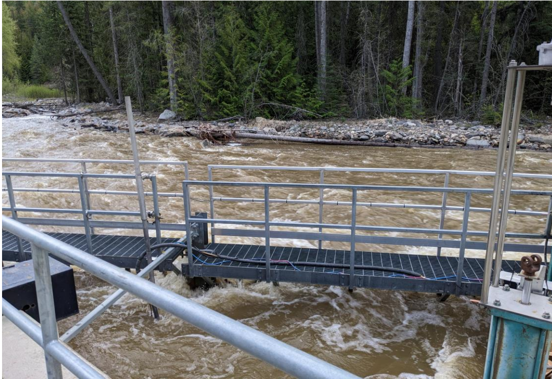
Turbidity in Mission Creek, May 5 – Raw Water at Intake Site
