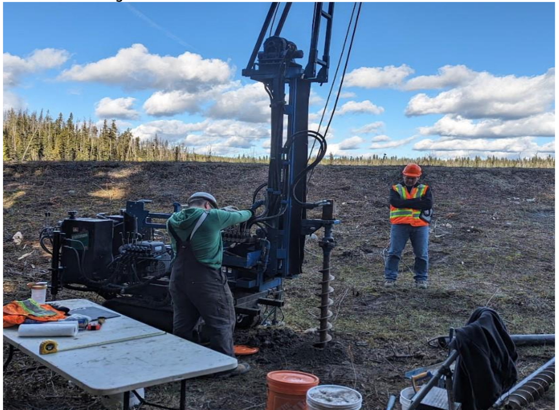
Geotechnical drilling at James Lake Dam
