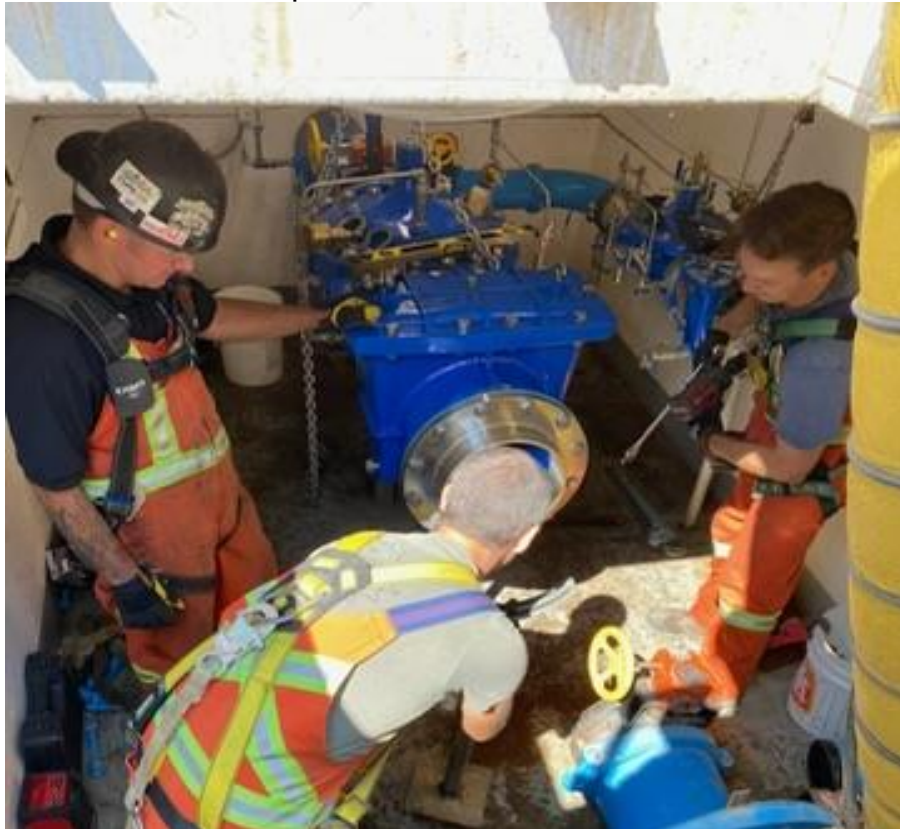
PRV #15 Control Valve replacement
