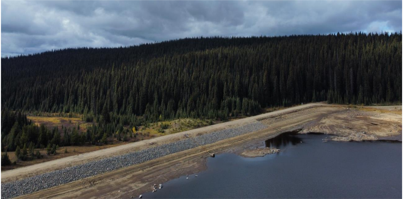
Fish Hawk Dam rip-rap project
