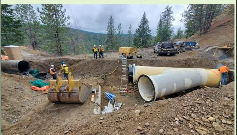
Work at the west portal of the future tunnel is shown in the photo. This connection has large diameter butterfly valve in place that will allow future tunnel extension work to be carried out with uninterrupted service to BMID water supply.
