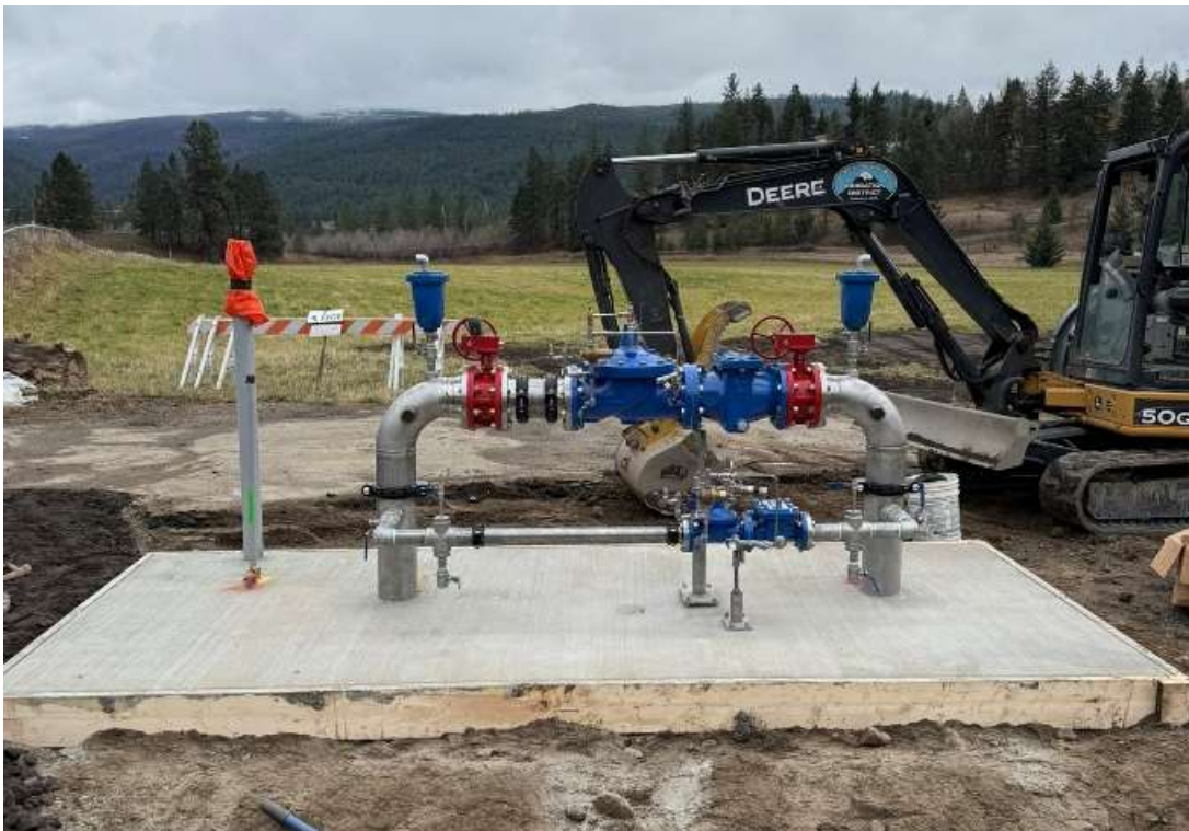
PRV #29 under construction
