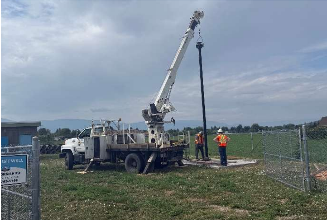
1965 Cornish test well decommissioning
