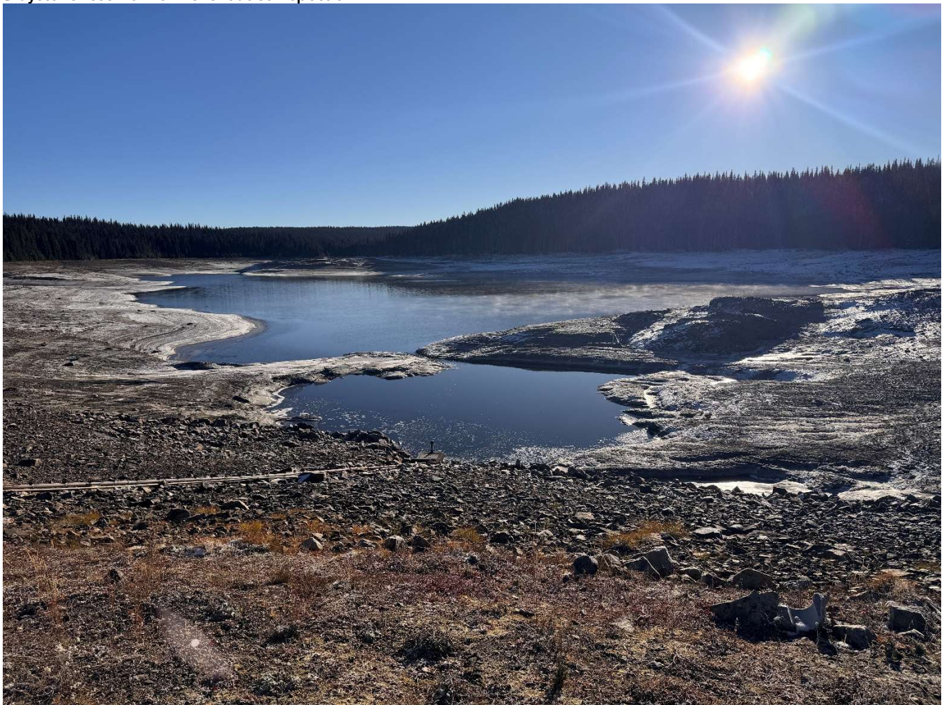
Graystoke reservoir low level outlet inspection
