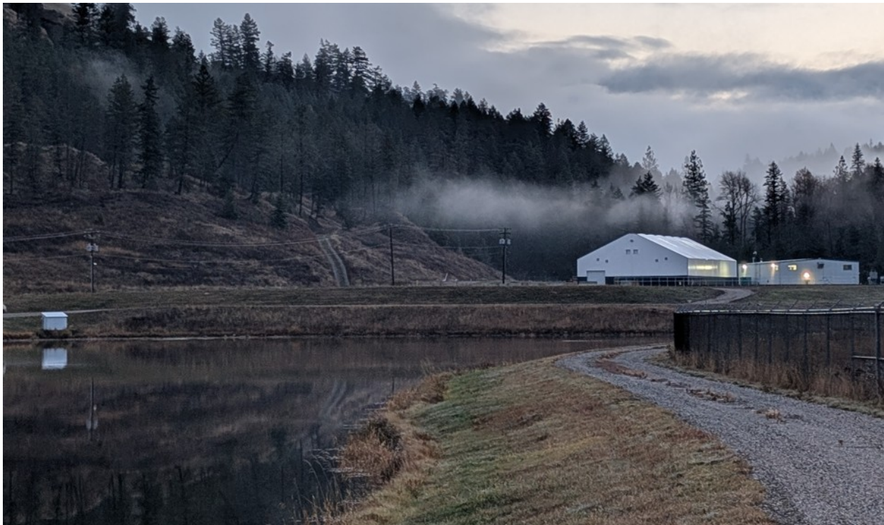
Stevens Reservoir – after Water Treatment Plant clarification
