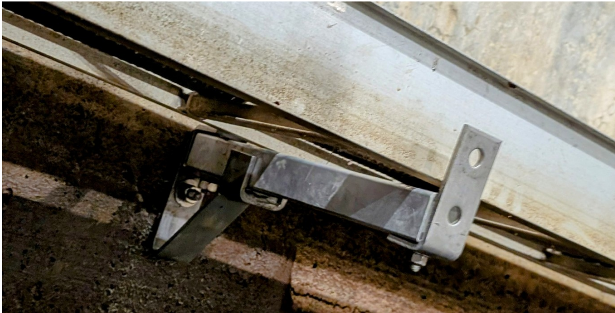
Stainless steel bracing added for electrical conduit trays
