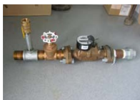
50mm meter assembly with meter, isolation valve, blow-off assembly
